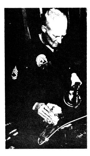
Figure 4-5. Heating pine tar with a blowtorch.
